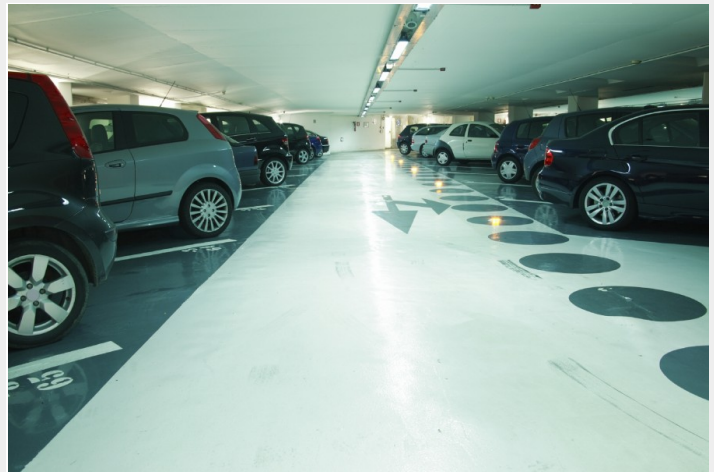
Parking Garage FACING NORTH
