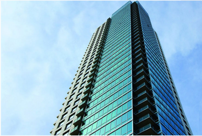
Exterior Entrance FACING SOUTH
