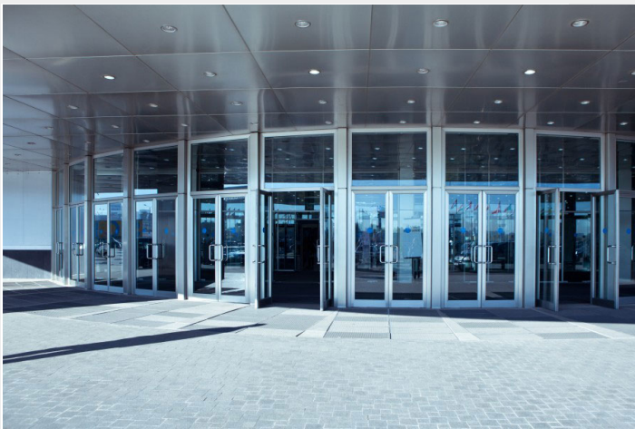
Exterior Entrance FACING SOUTH
