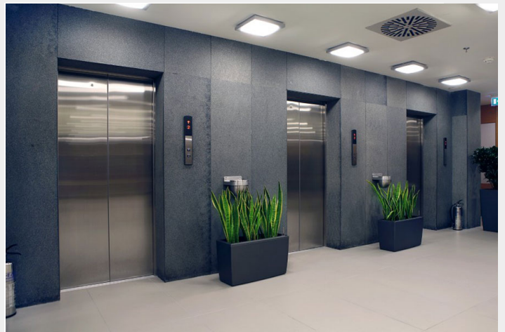
Elevator Bay FACING SOUTH
