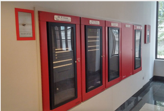
Life Safety FACING EAST
